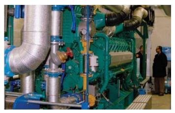
A 1.5 MW lean-burn gas generator set provides heat and power as well as  $CO_2$  to accelerate the growth of tomatoes at a large greenhouse in Belgium.
