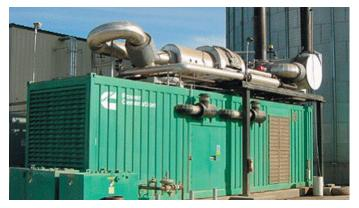
This cogeneration unit produces 1,250 kW of electricity, 2,200 pounds of steam and 30 gal/min of hot water, while besting local air-quality standards at a California animal feed processor.
